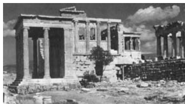
Athens, Akropolis, Erechtheion from the west
