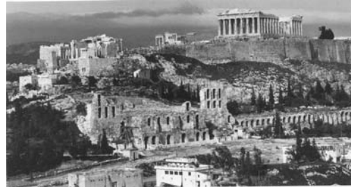
Athens, Akropolis, View from the South West
